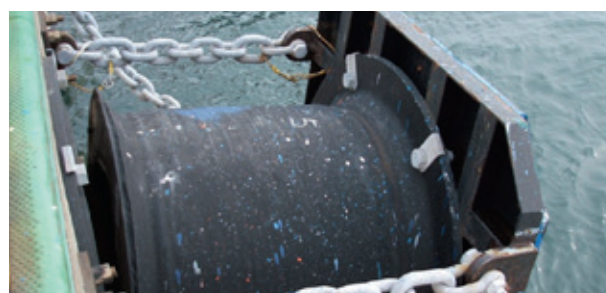
Insufficient bonding
